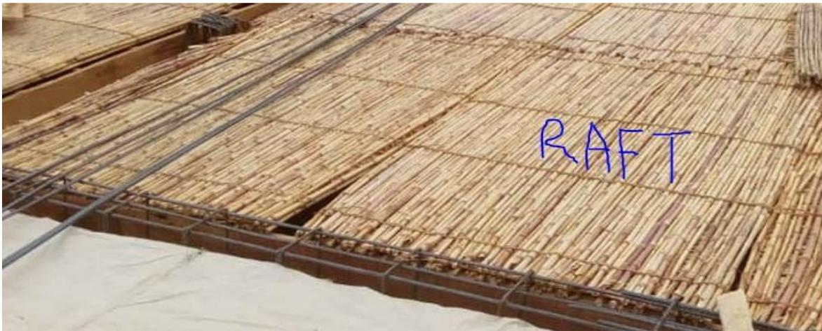
**Figure 1.** Sorghum raft placed as soffit in suspended slab construction.
