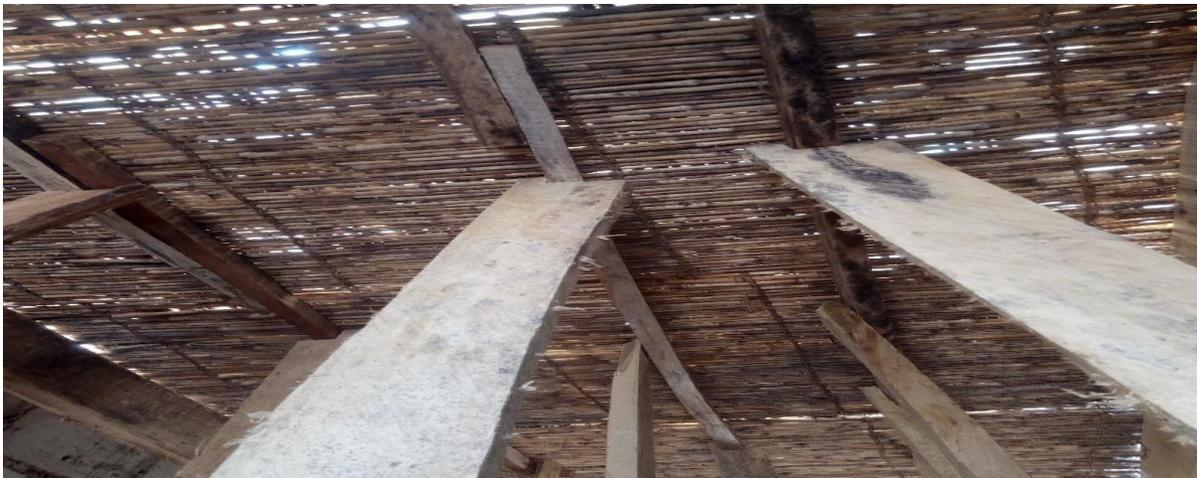
**Figure 2.** Underside of sorghum stalk soffit.
