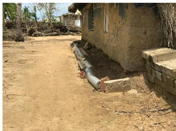
Fig. 9: Concrete-filled 4inch Pipes Around Building (Source: Author's Photograph)
