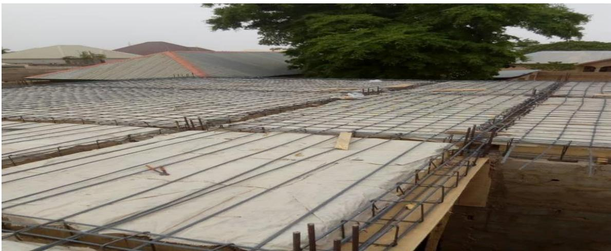
**Figure 5.** Arrangement of reinforcements on soffit formwork.
