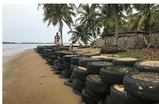
Fig. 7: Car Tyres Filled with Concrete (Source: Author's Photograph)
